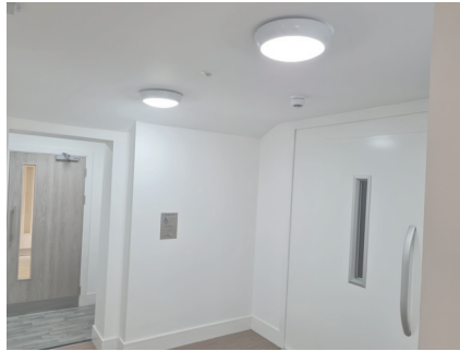
CCECO Luminaire corridor installation.
